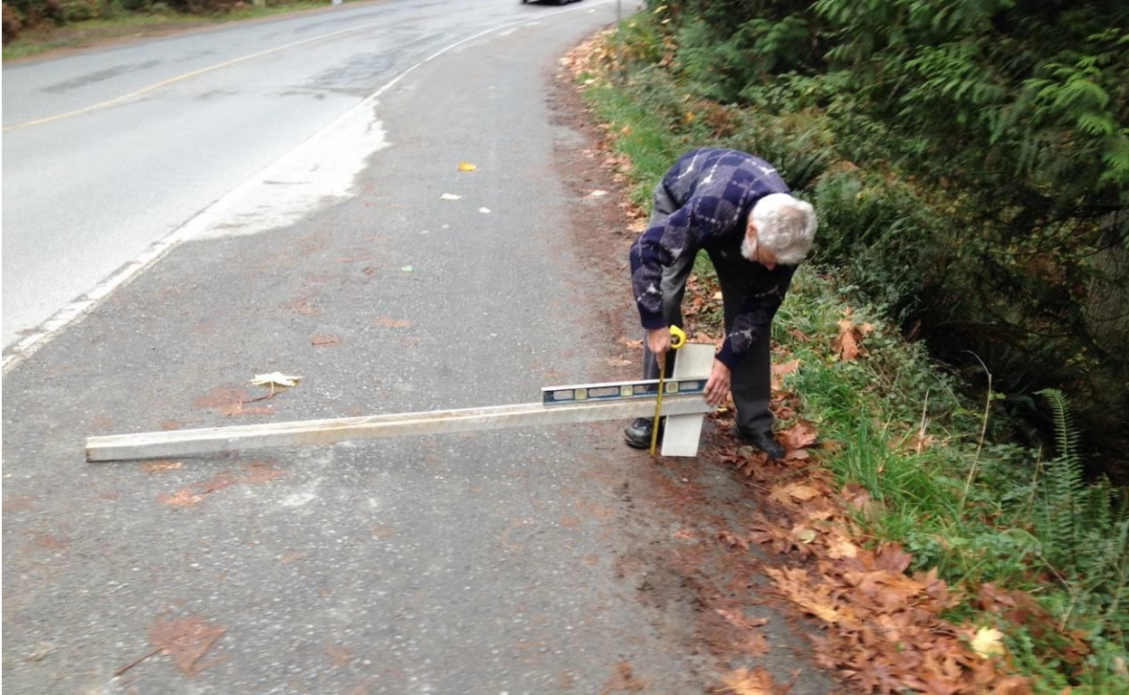
Measurements of the slope of the road shoulder in the ferry queue lane at the southern end of Taylor Bay Road (Submitted by Jeremy Baker)
